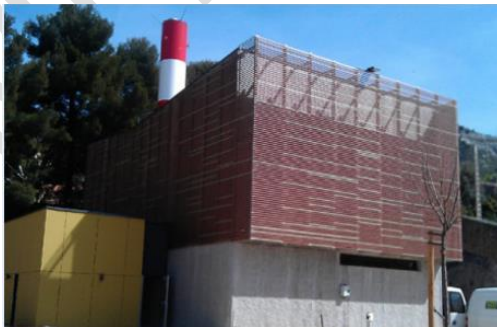
Figure 49 Chaufferie biomasse îlot Sainte-Anne
