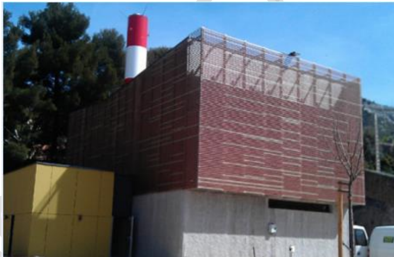
Figure 34 : Chaufferie biomasse îlot Sainte-Anne
